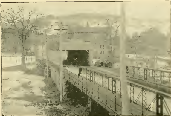
Wooden Bridge at Thomaston, Recently Demolished.
